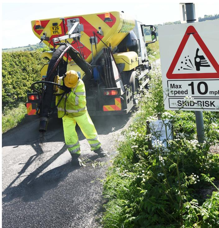
Spray injection machine in use
